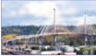
Port Mann Bridge, Vancouver, British Columbia
