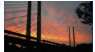
Eleanor Schonell Bridge, Brisbane, Australia
