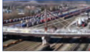
Coast Meridian Overpass, Vancouver, British Columbia
