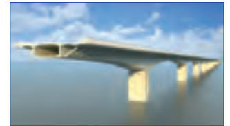
Ganga River Bridge, Bakhtiyarpur, India
