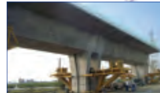
Taiwan High Speed Rail, Contract C295, Taiwan
