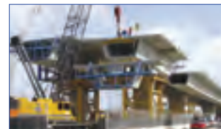
PR-181 Bridge, San Juan, Puerto Rico
