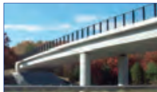
DCR Access Road, Randolph, Massachusetts
