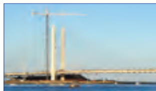
Indian River Bridge, North Bethany, Delaware
