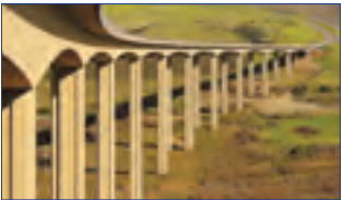
Otay River Bridge, San Diego, California
