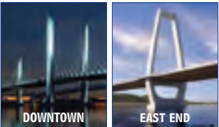
Ohio River Bridges Project, Louisville, Kentucky
