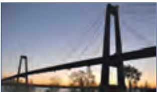
Hale Boggs Memorial Bridge, St Charles Parish, Louisiana
